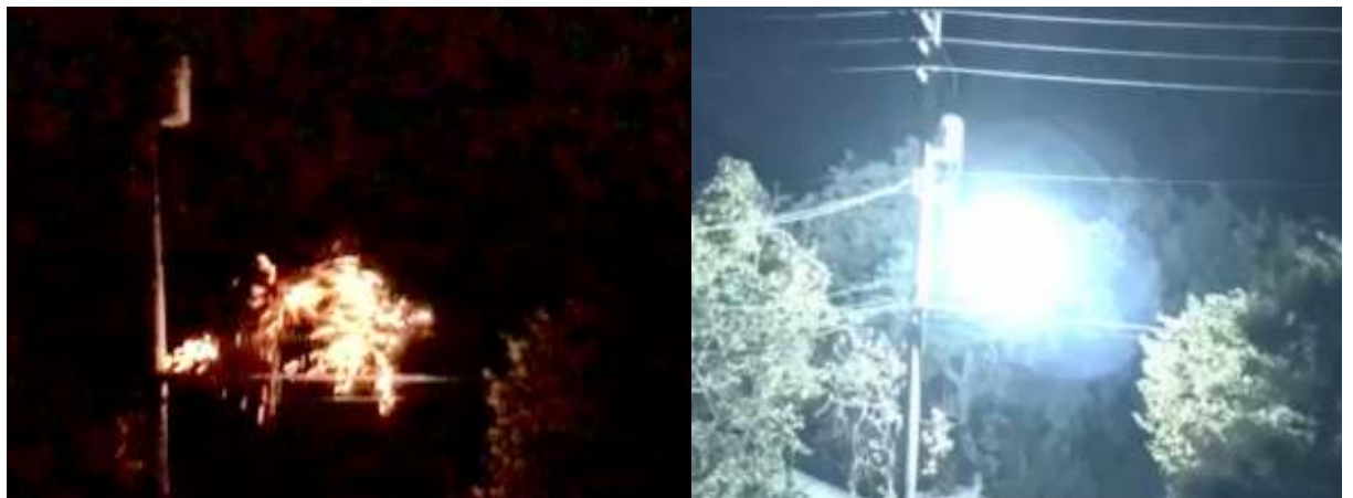
18 19 20 21 22 23 24 25 PG&E Electrical Equipment Sparking in Trees Near the Tubbs Fire 9
